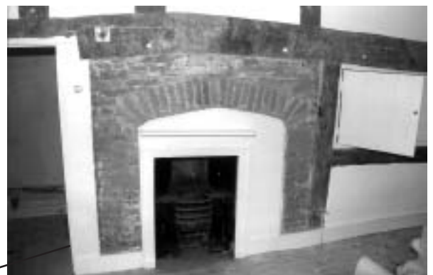
Tudor / Elizabethan fire place / chimney in timber frame
