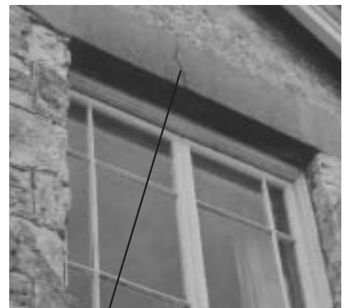
Cracked lintel
