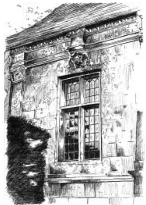
A mullion / transomed stone window with iron frames and lead lights.
