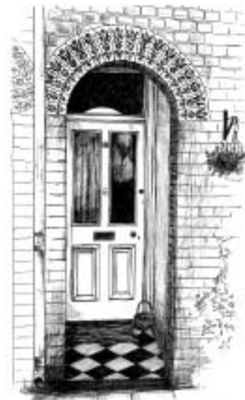
A well proportioned Victorian door with fanlight and glazed upper panels.
