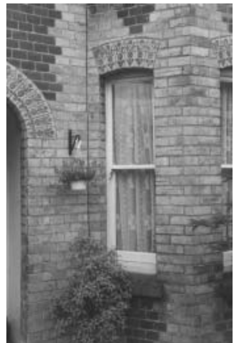
A late Victorian sliding sash part of a bay window. Note decorative horns, locally these are post 1870.
