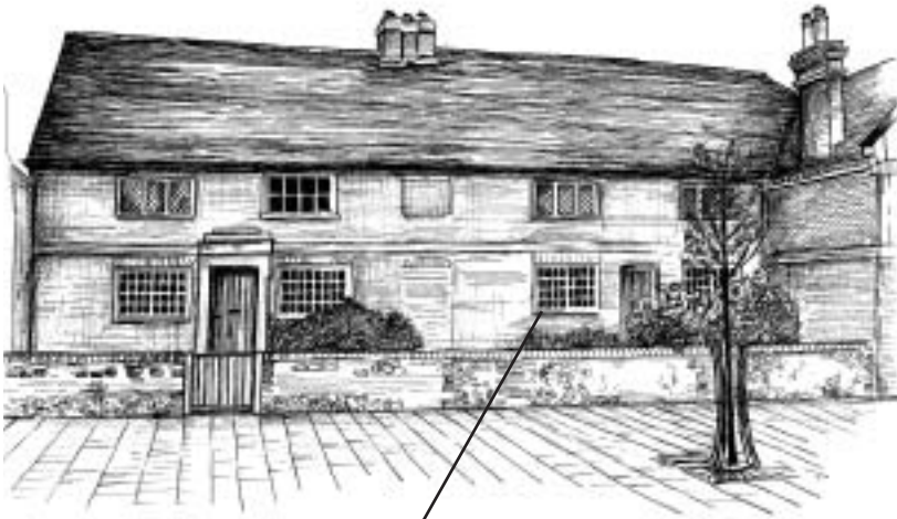
Horizontal sliding sashes can be found too.
