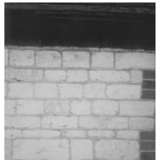
A well laid local malmstone wall with banded coursing using large bonding stones after 6 or 5 narrower courses.
